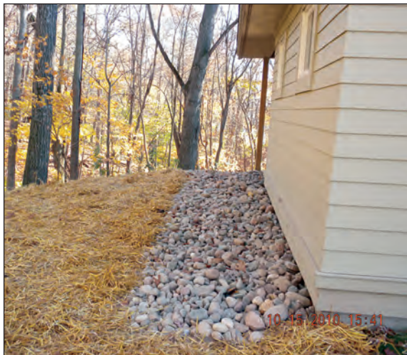
Diversion and rain garden design at Bone Lake's north landing.
