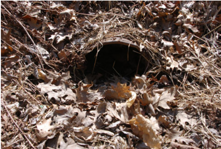
Culvert #7 w/sediment deposition is improperly sized.
